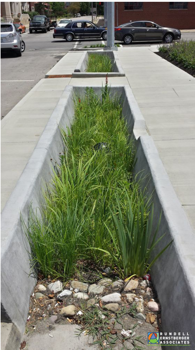
Figure 4: Rain gardens can help prevent flooding on roads. (Source: Rundell Ernstberger Associates)
